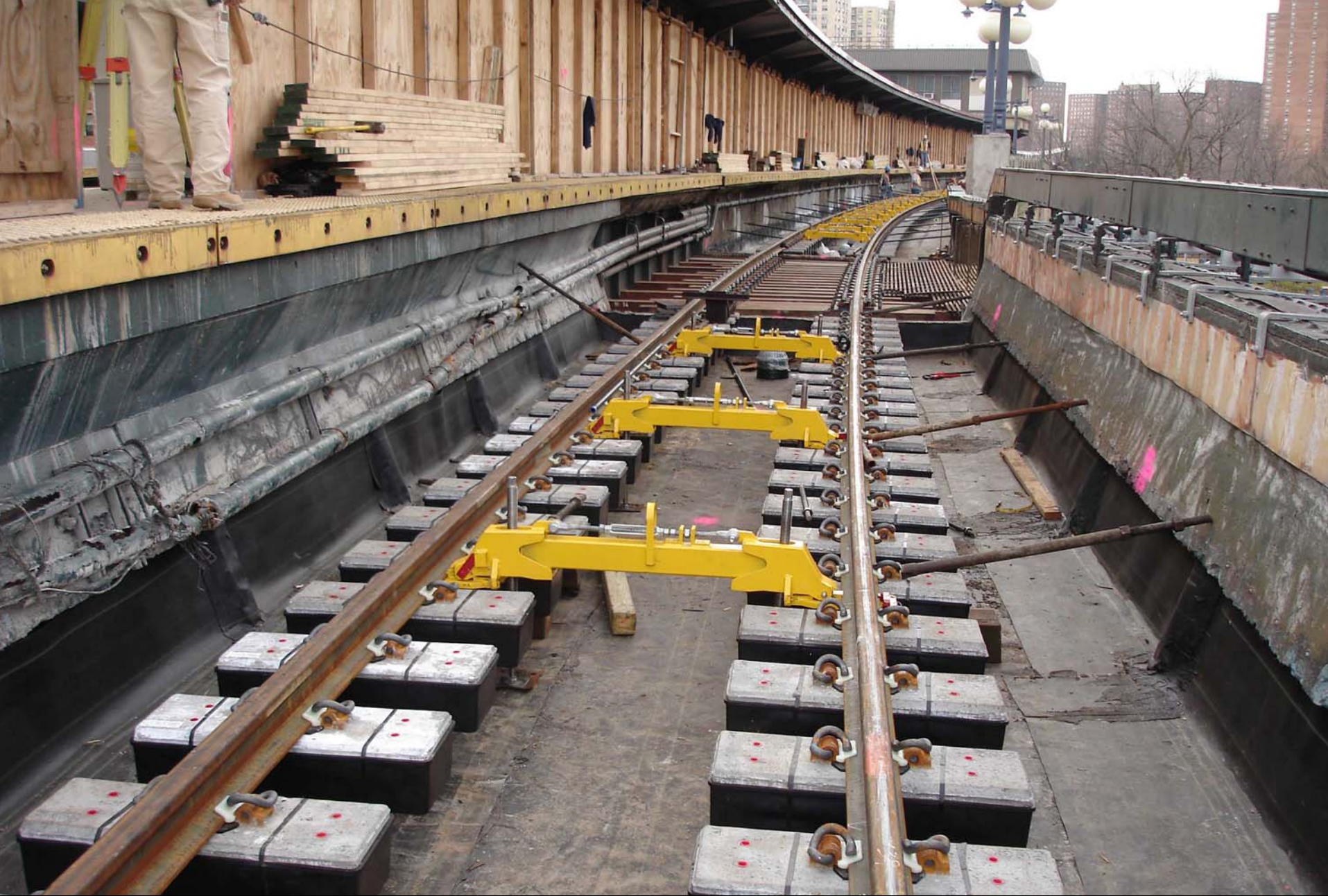
Installation of New Low-Vibration Track at Ocean Pkwy. Station
