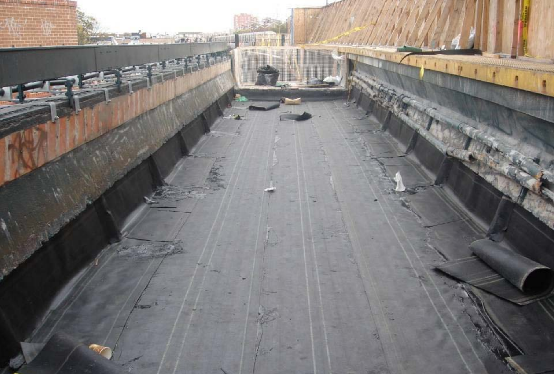
Installation of Deck Waterproofing at Ocean Pkwy. Station
