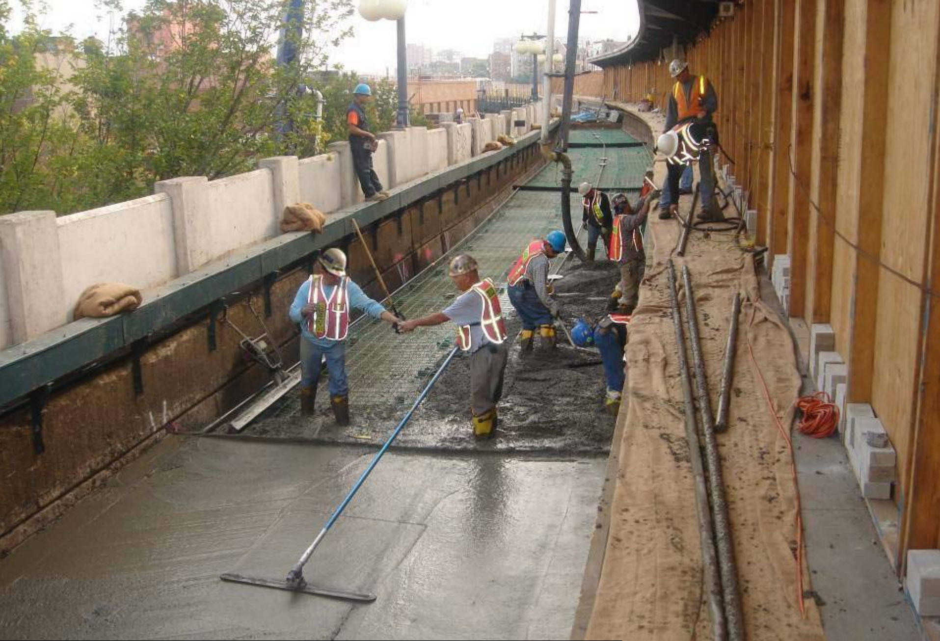
Installation of Deck Slab at Ocean Pkwy.
